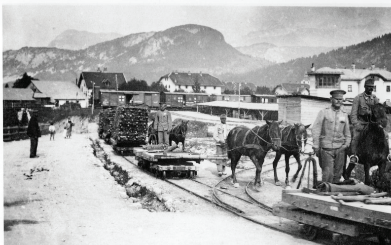
Figure 3. Narrow gauge horse-drawn railway, 1915–1916. The horse-drawn railway was the first section of the hinterland supply system, which ran from the train station to the eastern end of Lake Bohinj. Courtesy of the National Museum of Contemporary History, Slovenia.
