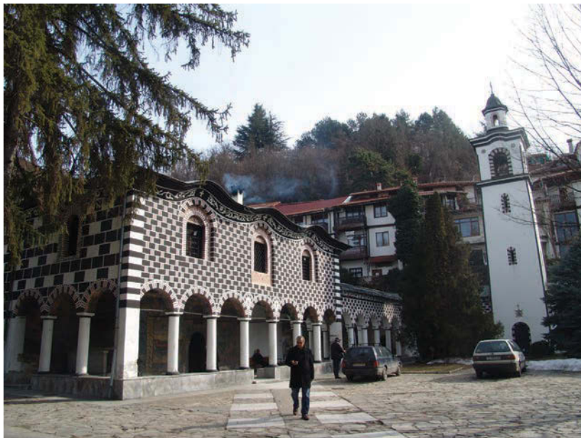
Figure 2. 'Presentation of the Virgin' Cathedral in Blagoevgrad (FtAIF No. 1581, arch. unit 18).
