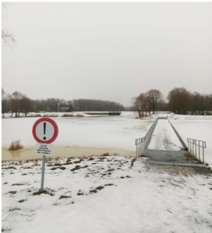
Figure 6. Recreational trail bridge at the Lubana wetland TIC. Photo by Karlis A. Konkovs.
