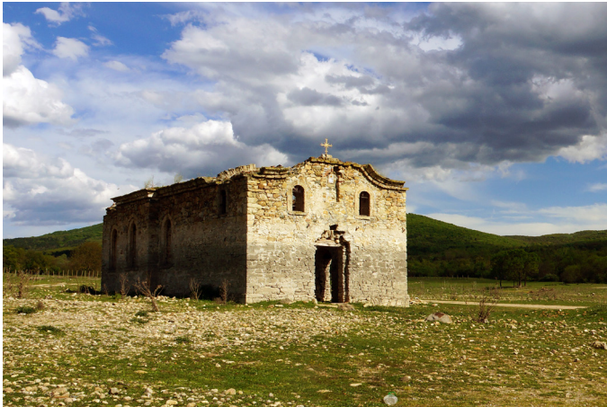
Figure 1. The Submerged Church “St. John of Rila” at the Zhrebchevo Reservoir. Photographer: Yana Gergova, 2.05.2019
