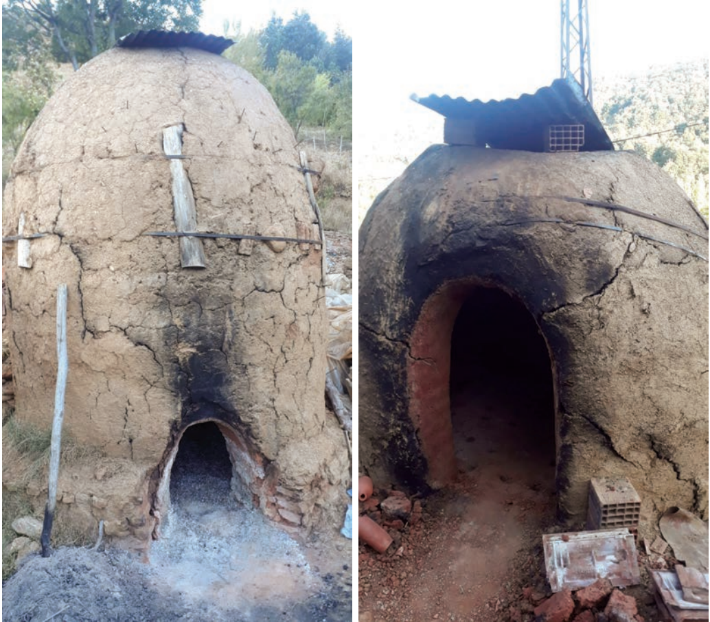
Figure 22. Doğanhisar pottery kiln, “Ateşlik” (fire box) on the left, the mouth of the product filling on the right.
