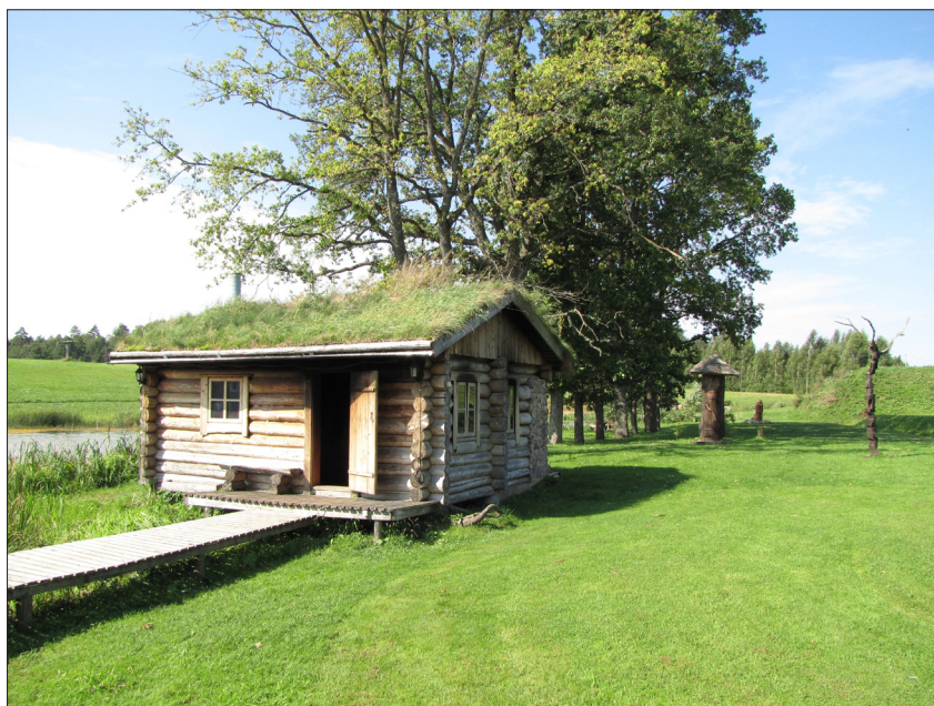
Figure 3. The newly built smoke sauna in Nõiarik (Sorcerer's Kingdom in the Primeval Valley of Lake Uhtjärvi), Urvaste municipality. Photo by Helen Sooväli-Sepping 2010.
